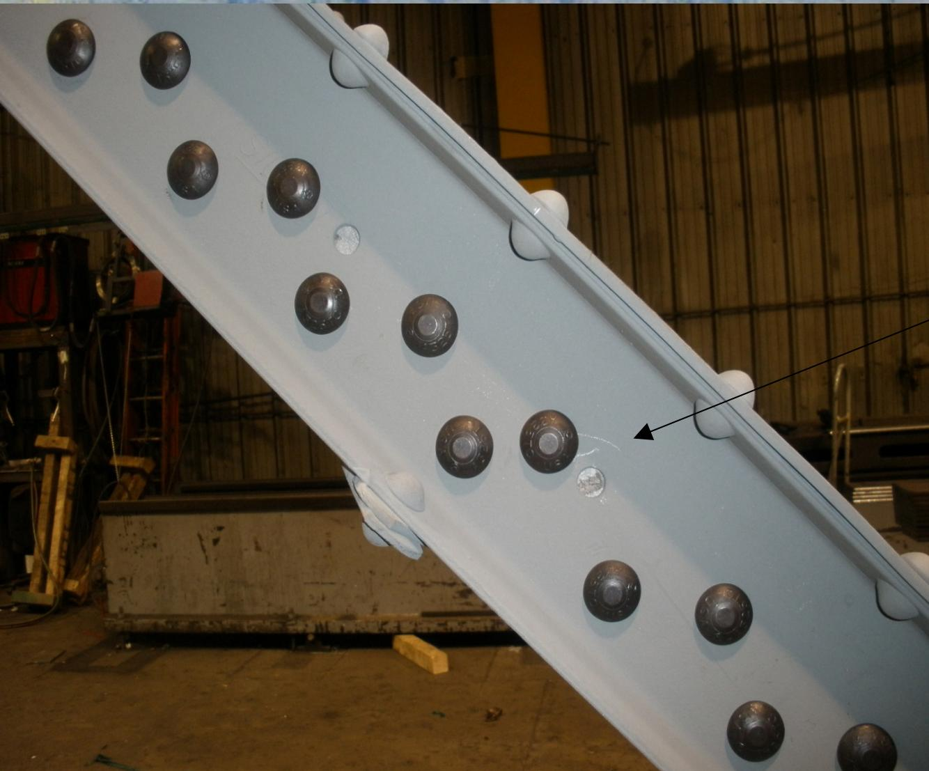
Original end post and top chord members were reused and strengthened where required. New bolts were domed headed to match shape of rivets.
